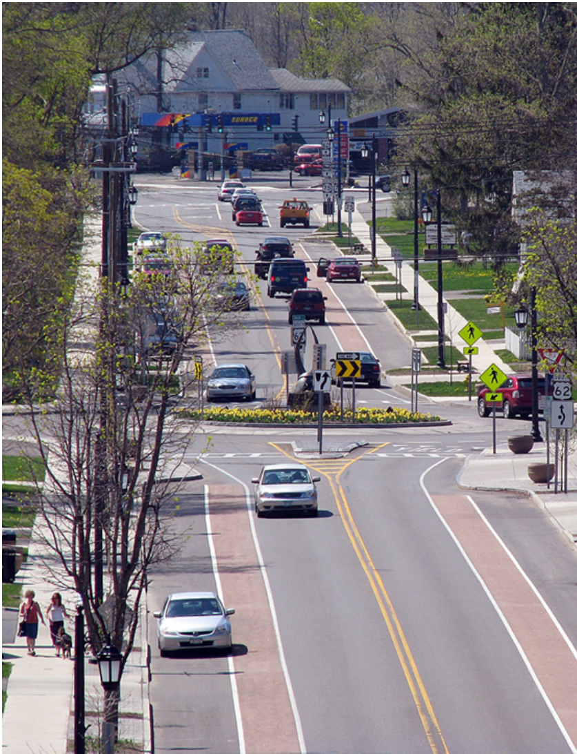
The Route 62 road diet project in Hamburg, NY demonstrates how state highways may function as walkable mixed-use environments. The brick-colored areas on either side are not formal bicycle paths but provide some haven for cyclists and slow traffic. Photo Credit: NYS DOT
