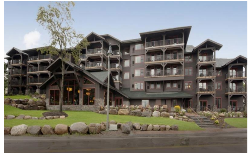
The Hampton Inn & Suites at Lake Placid is a good example of a national brand altering their standard brand prototype to better fit the rural character of a community with an established identity. Photo Credit: Regional Office of Sustainable Tourism/Lake Placid
