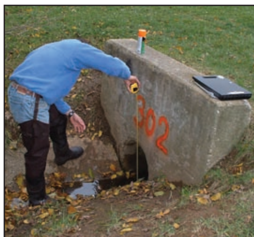
Figure 27: Measuring Outfall Diameter
